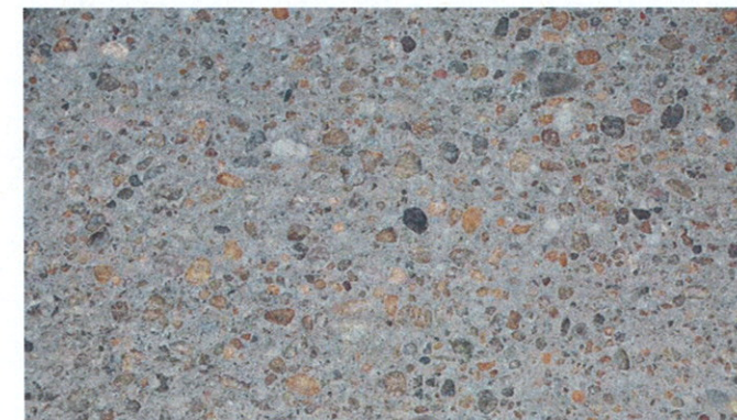
SHOT BLASTED CONCRETE PAVING
